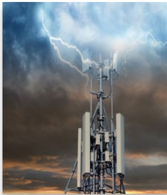
Strike at base station tower
