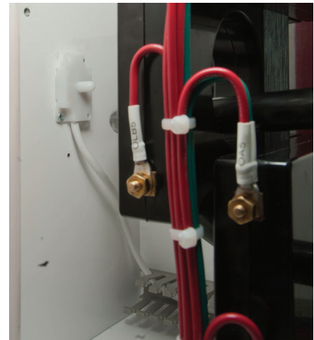
Examples of appropriate point sensor installation.
